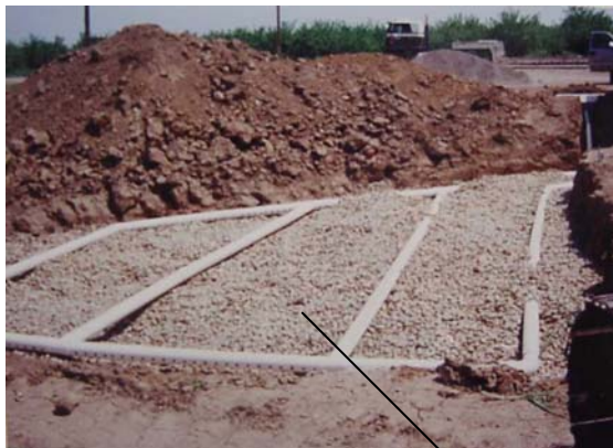
Double Walled 5' each way when crossing water line.
