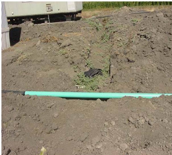
Double Walled 5' each way when crossing water line.
