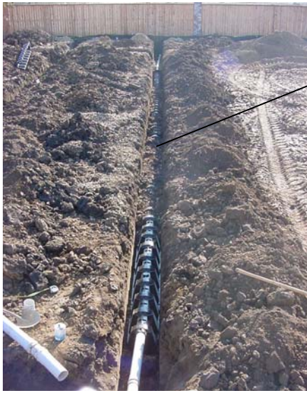
Hand shovel & compact soil around chamber to 2" above chamber.
