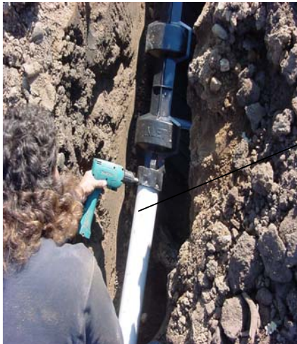
Sheet Metal Screw, 3 per connection
